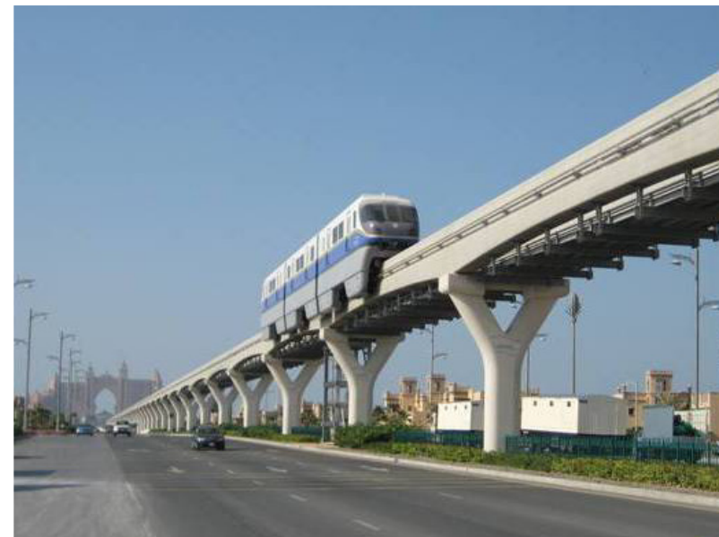
Dubai Monorail (under construction)
