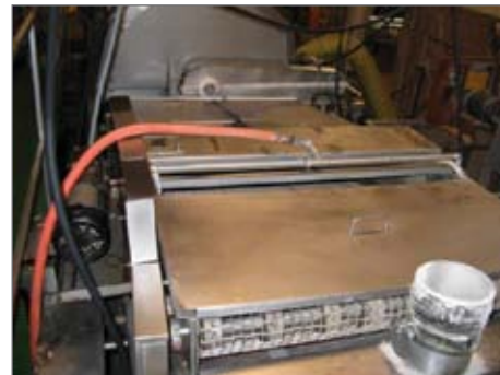
Compressed air pressure dewpoints must be below -15 °F (-26 °C) to inhibit the growth of fungi and microorganisms in the piping system.
