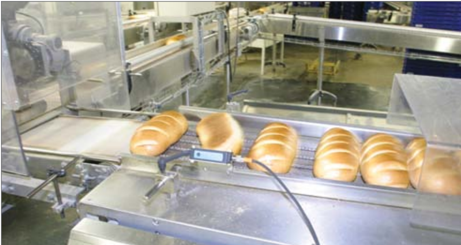
Compressed air is used to blow crumbs off of bread in a commercial bakery.
